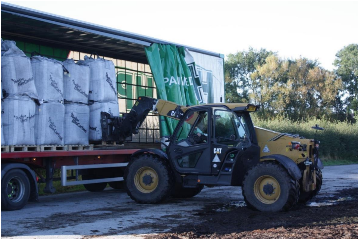
Figure 46. Biochar was delivered to site by HGV in palletised bulk bags. Bags typically contained 400-455kg biochar. Full trailer load was c. 20t.
